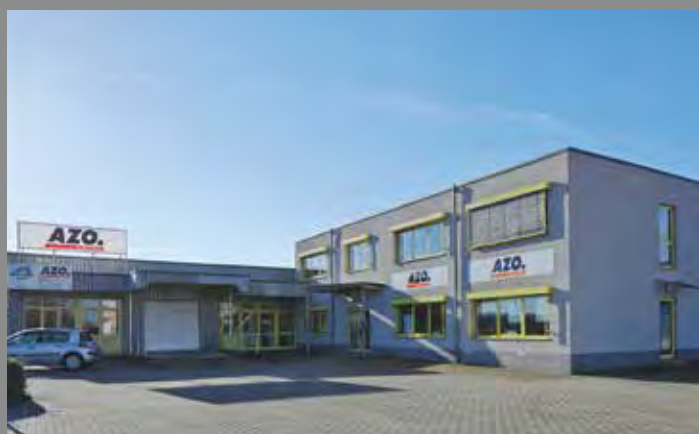
AZO LIQUIDS office building
